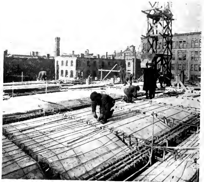
Floor view showing reinforcement for main trusses, beams and slabs.
